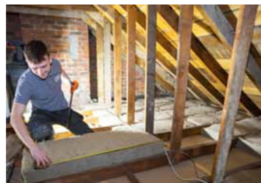
IndiNature insulation batts being installed.
